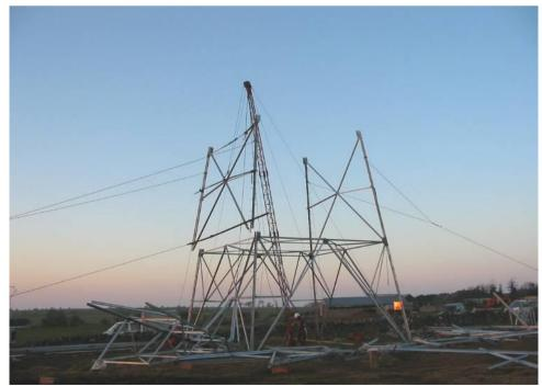
Figure 6.3 Derrick pole at tower base
