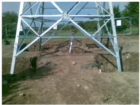
Figure 6.6: Photograph of steel tower base in open excavations.
