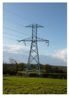
Figure 3.3: Typical steel angle structure
