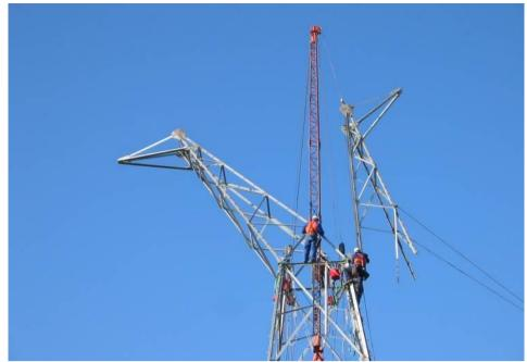
Figure 6.4: Lower part of the tower head being dropped into position
