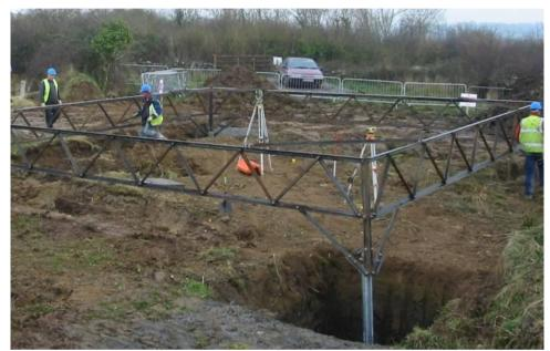
Figure 6.2: Photograph setting template being prepared for final concreting
