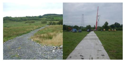
Figure 5.1: Temporary Stone and Aluminium Panel tracks
