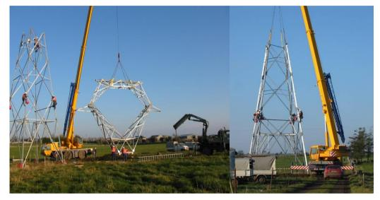
Figure 6.5: Tower erection by mobile crane
